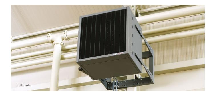
Jaga's unit heater features technology generates powerful airflow with even temperature distribution. By reducing the return temperature, the unit heaters are able to reduce stratification and the amount of cold air build-up at the ground level. This means shorter operational times and greater energy savings.
